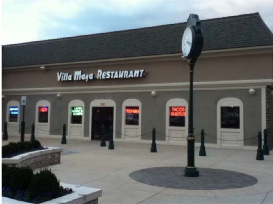
Villa Maya Restaurant 5532 Norbeck Road Rockville, MD 20832 Located in the Rock Creek Village Center
